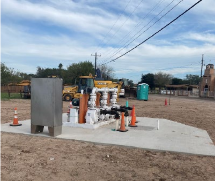
Rio Grande City, Texas installed a new Lift Station with backup pump at their facility in 2019
